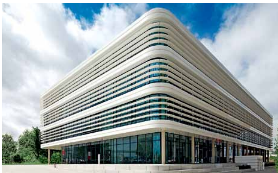
© Depenbrock Systembau, Bielefeld
